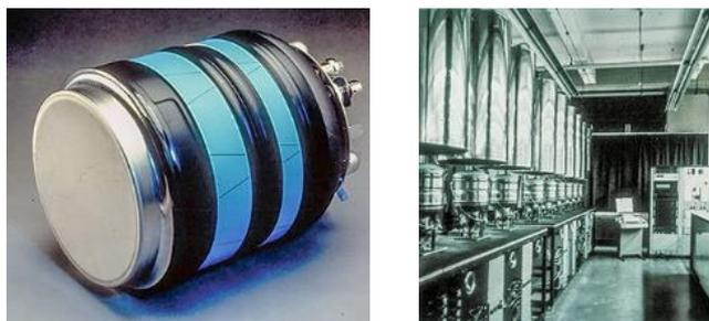
Analog video was introduced in the 1960s. This development removed a major limitation on the position of the operator relative to the patient (FIG 36). As a bonus, everyone in the room (including the patient) could see the fluoroscopic images. It also enabled the development of remote-control fluoroscopes with the image intensifier under the table (Figure 37). Placing the image receptor under the table results in having the X-ray tube over the table. The irradiation of an operator's eyes is
